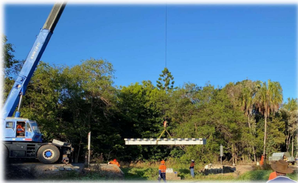
ASCR trades along with KWIK LIFT get ready to bolt down this section into place on the concrete abutments.
